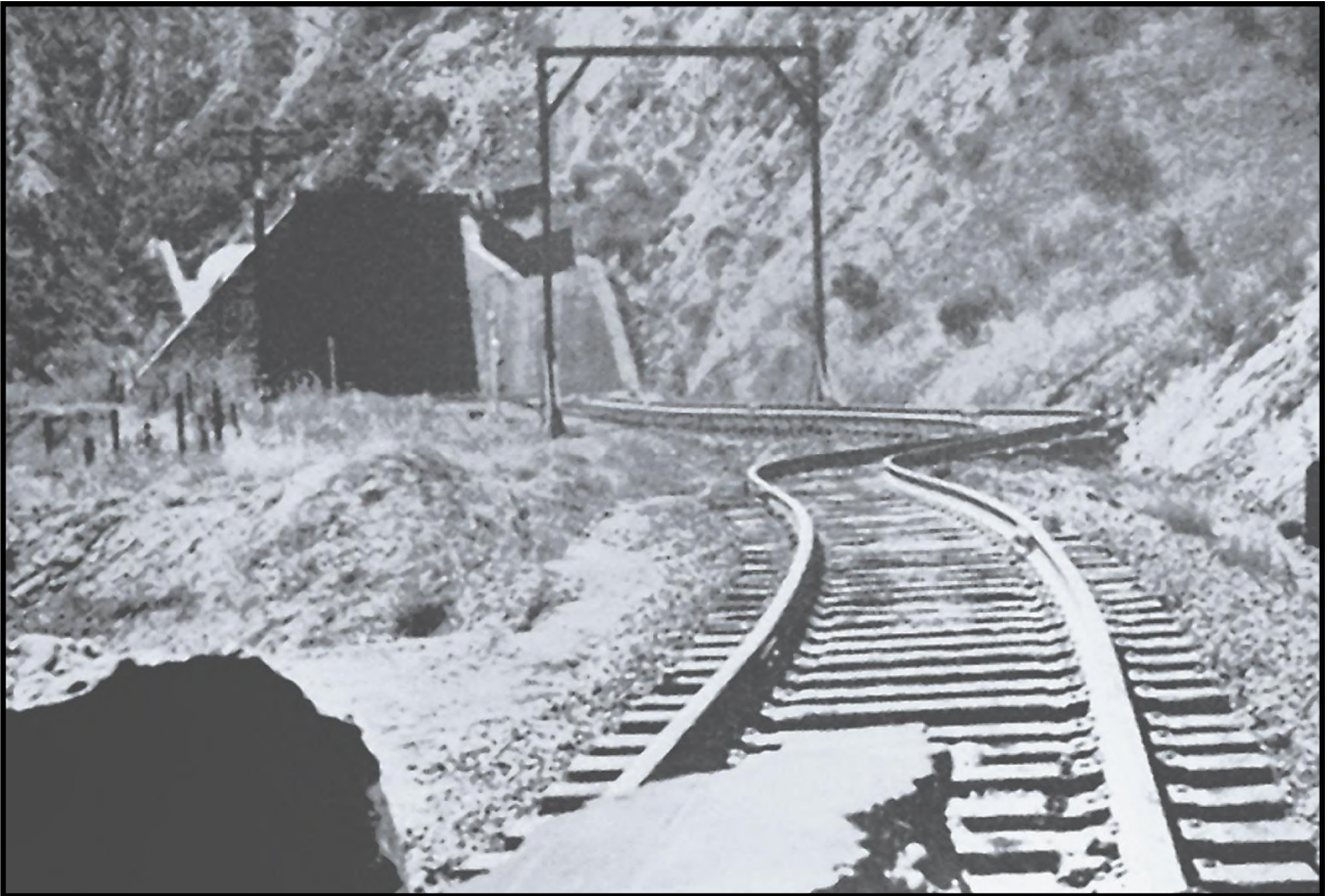
Seismic ground faulting buckled tracks at several locations including inside tunnels in the 1952 earthquake south of Bakersfield.
