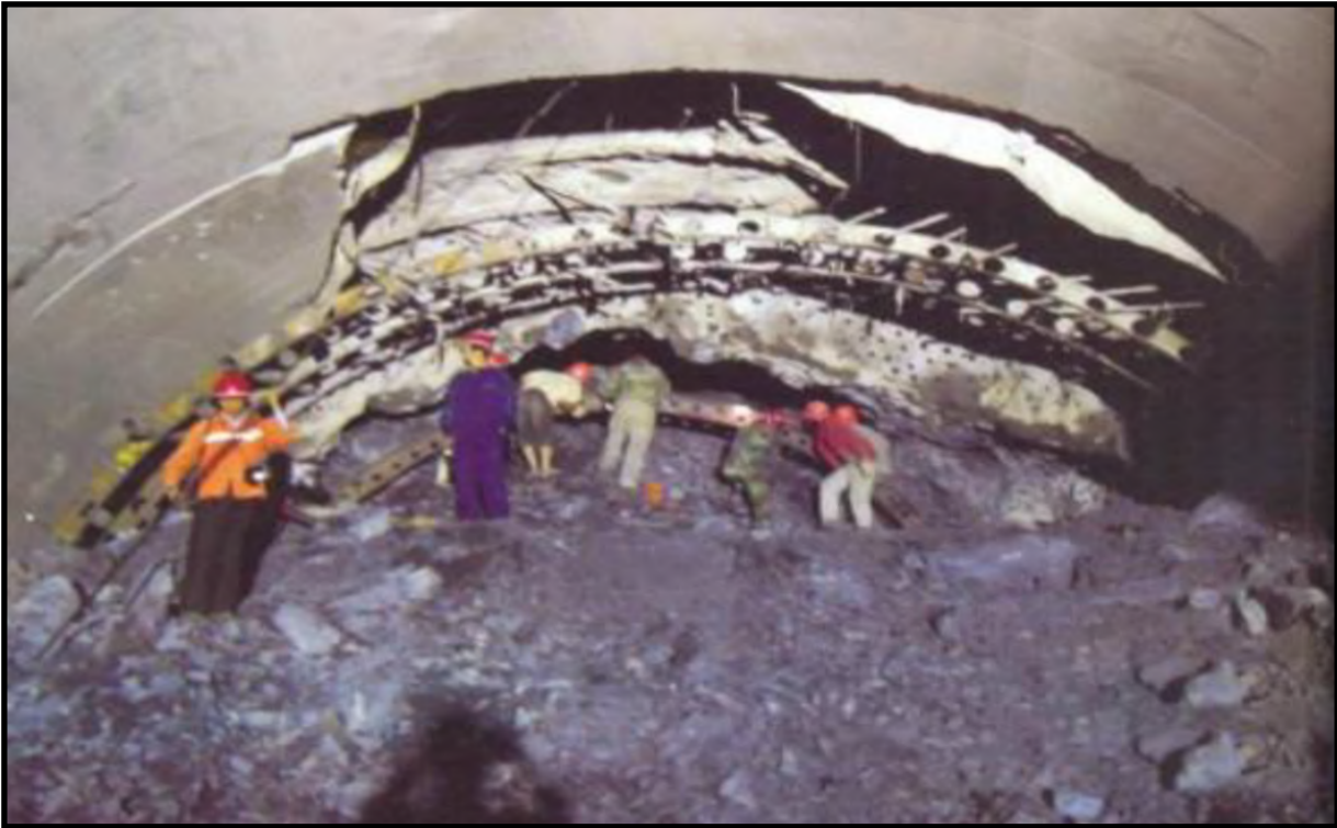
Wenchuan earthquake 2008 tunnel collapse at fault crossing.
