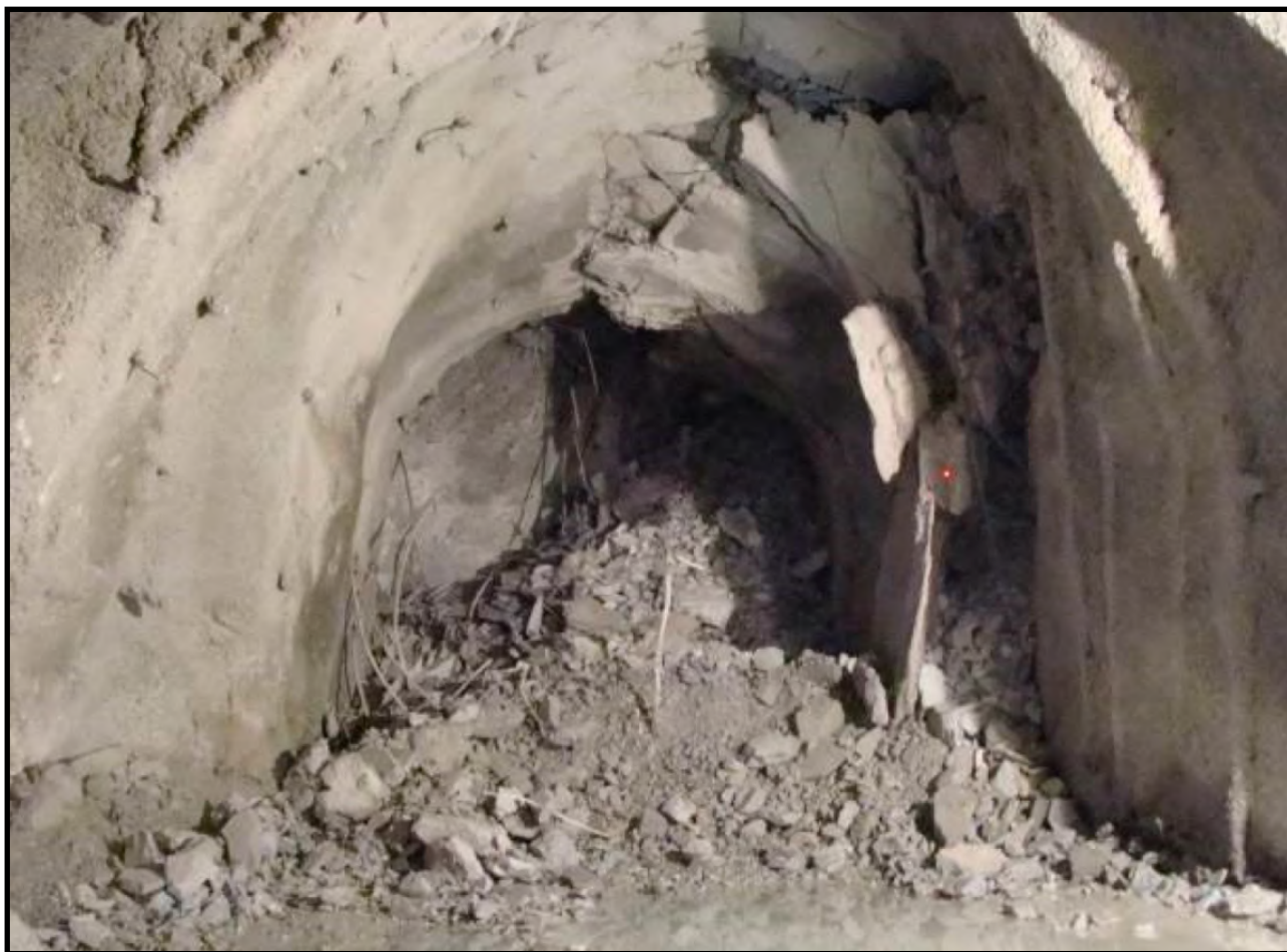
Rock burst in a Chinese tunnel
